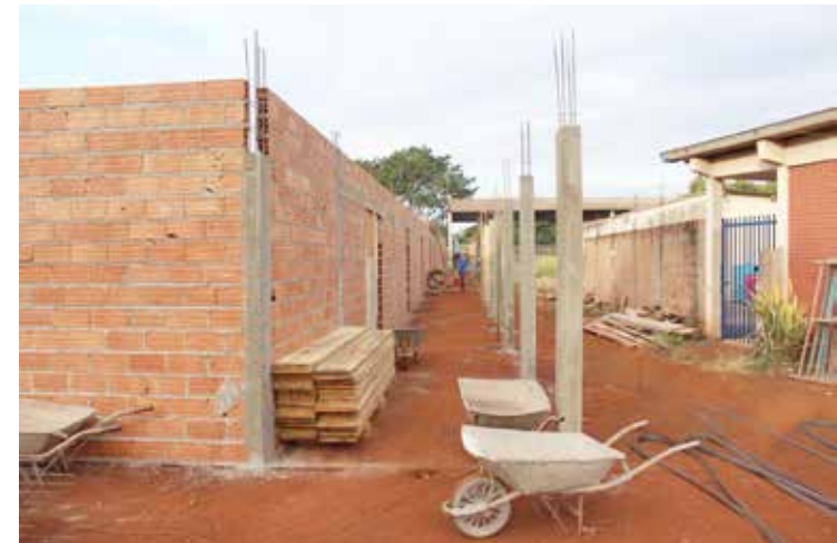
Obras na Escola Municipal Rotary Club
